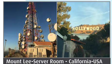
Mount Lee-Server Room - California-USA
