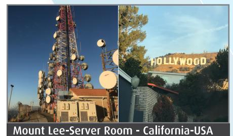
Mount Lee-Server Room - California-USA
